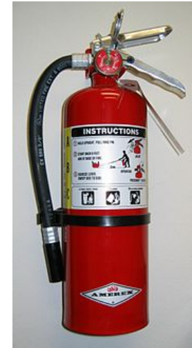
UMMC maintains 10lb Extinguishers A, B, and C.
